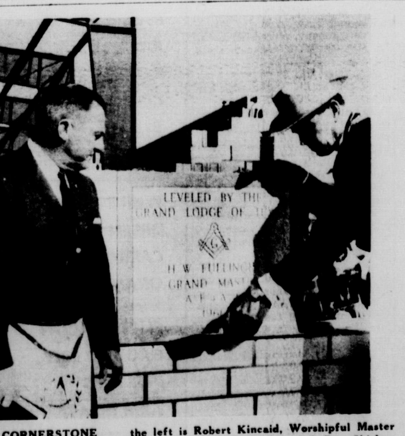
GRAND MASTER LEVELS CORNERSTONE H. W. Fullingim of Odessa, Grand Master of Masons in Texas, is pictured on the right as he levels the cornerstone of the new building under construction at the Crowell School. On
