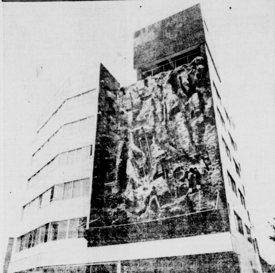
An imaginative Japanese manufacturer of mountain climbing equipment has created on one facade of his new building in the heart of Tokyo a 65-foot replica of an 84-degree rocky slope. The "Tokyo Rock" was designed by rock-climbing experts and affords supervised training for neophytes as well as exercise for the more seasoned climbers at a cost of 65¢ per hour. As a precautionary measure, there is a safety net along the lower ledge. The simulated slope extends from the second floor to the roof of the six-story building.
