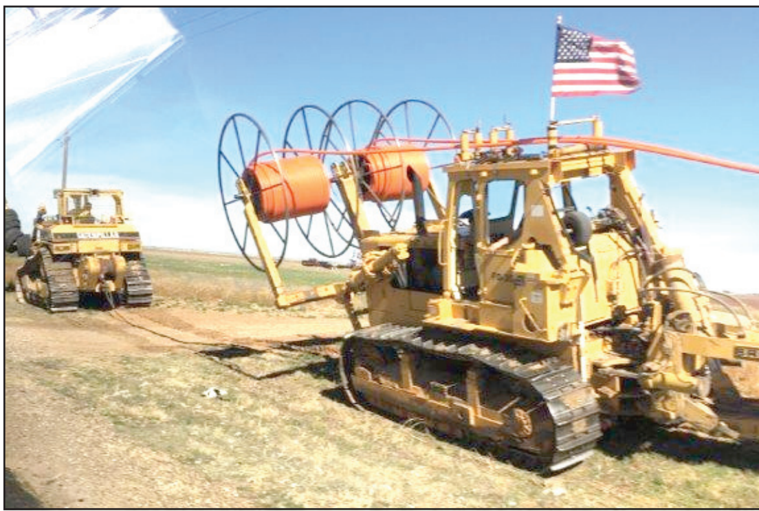
PLOWING IN DUCT --Adorned with a US flag and two large reels, a crawler tractor operated by a contractor plows in part of 78 miles of protective duct installed in West Texas Rural Telephone Cooperative's Oklahoma Lane, Parmer, Tharp and Hub rural exchanges of Parmer County, with fiber optic cable injection to follow in the future. (Photo by Raquel Vallejo)
