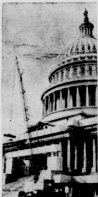
NEW LOOK —East front of the nation's Capitol building is covered with scaffolding as preparations go forward to extend the building forward some 32½ feet. Purpose: more room for the solons. Present sandstone facade will be duplicated in marble when the extension has been completed.
