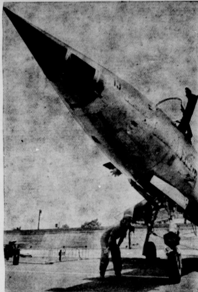
NOSING SKYWARD —As sleek as a sharpened pencil point, the nose of a Republic P-105 Thunderchief towers over test pilot Carl Ardrey at Farmingdale, N.Y. The pilot is studying a new steering device built into the nose wheel of the Air Force supersonic fighter-bomber.
