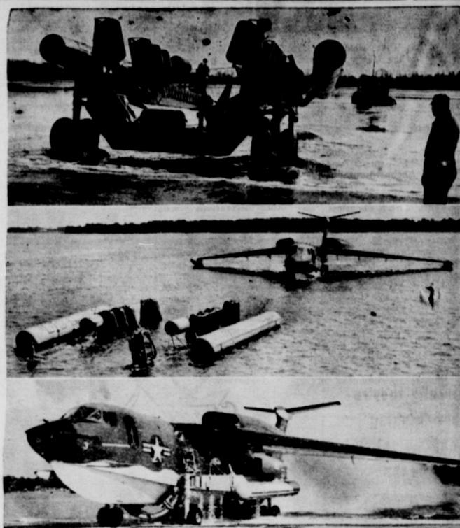
**TAXI ASSISTS TAXI**—Unlike a fish out of water, this big Navy P6M Seamaster gets a terrestrial taxi ride from a newly developed beaching vehicle at the Martin Company's Ballinger seadrome. Top photo shows the device ushered into the water. The Seamaster, center photo, heads for the floating taxi whose hydraulic pads will grasp the plane's hull. On land, bottom photo, the P6M, nestled in the beaching vehicle's cradle, taxis under its own power.
