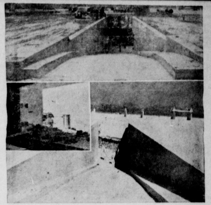
AUTO ENTRANCE ramp burrows inconspicuously into the desert as it leads down to a dual-purpose underground shelter and garage at the Operation Plumbbob atomic tests in Nevada. Lower photo shows how the A-bomb blast crumbled part of the concrete retaining wall but failed to block the entrance. To the right of the crumbled wall is the entrance, closed by a 100-ton, four-foot-thick reinforced concrete blast door (inset), which was undamaged. (NTO Lookout Mountain Lab Photo)
