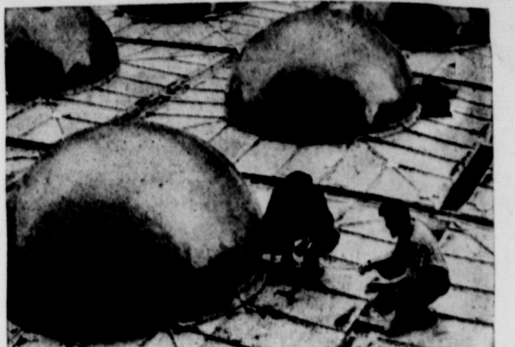
ONLY A ROOFTOP—This is only a rooftop—not a landing field for flying saucers. The huge, plastic "blisters" providing more daylight for people underneath in a Paris, France, banking establishment.
