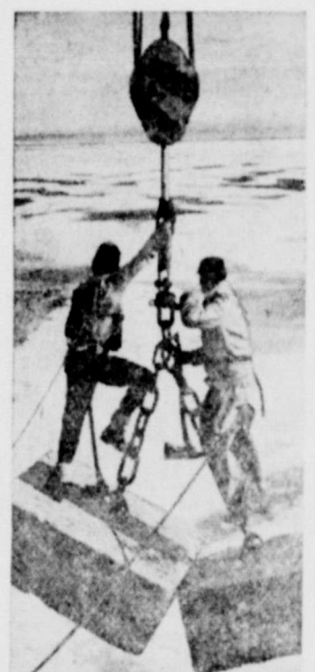
TRADITIONAL —A procedure used by early Arctic explorers to plow through heavy ice is utilized by crewmen of the U.S. Coast Guard cutter Spar as the ship steams along the route of the famed "Northwest Passage" across the top of North America. The men are lowered with axes on concrete blocks which serve a double purpose: weights to warp the ship free from ice and crushers to pound the ice to powder.
