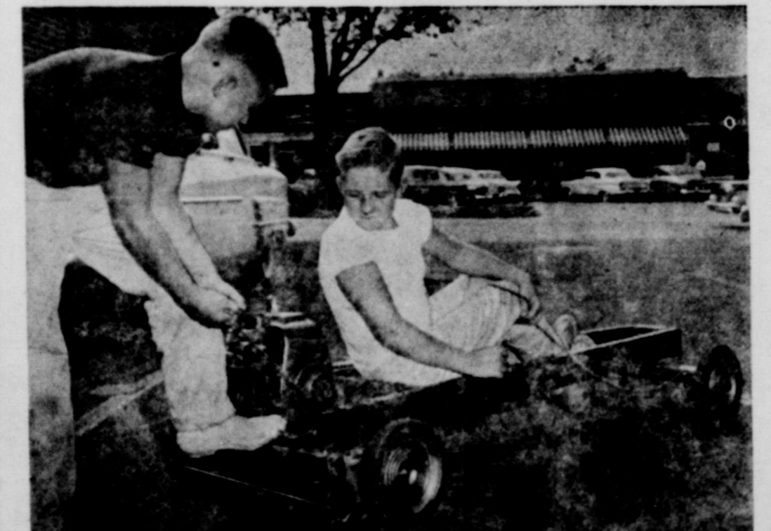
BUT DOES IT RUN? —The ultimate in stripped-down hot rods, this contraption, made of two-by-fours and one-inch boards, is readied for a small trip in Fair Lawn, N.J., by its builders. Peter Katz, 13, left, starting the engine, and Dennis La Huff, 14, bought the lawn-mower engine from a repair shop for $20 and spent another $15 to rig up the rest of the rope-steered vehicle. It'll do 15 miles an hour, but not on town streets. The kids have been warned to keep out of traffic and drive only in the park.
