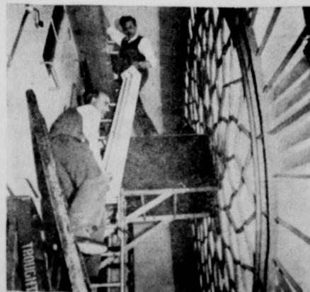
**LIGHT UP BEN'S FACE**—Behind one of the four faces of London's famed Big Ben, workers Eric Lucas, top, and Sid Harbour install one of the 56 fluorescent-type lighting fixtures which will illuminate the massive clock for the first time since 1954. The fixtures are replacing the ordinary electric bulbs previously used.
