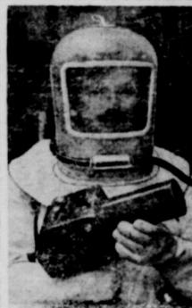
**NO LUNCHBOX?**—Here is a worker at the Mol, Belgium Center for Application of Nuclear Energy. Made of plastic with seams that zip together, the suit, designed to protect against contaminated air, is topped with a diver-type helmet. The worker breathes from a tank on his back.
