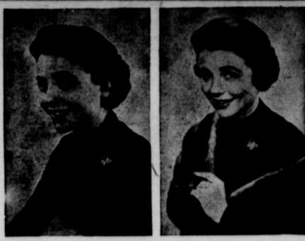
**FASHION NOTE FOR THE HARD-OF-HEARING.** A new Zenith Crest hearing aid can be worn ten different ways with any type of clothing. Left, the hearing aid in place—concealed by a rhinestone brooch and connected by cord to the earphone. Right, the wearer's hair hides the earphone. The Crest, a full powered 4-transistor instrument, weighs less than an ounce complete with battery. (H-A-D)
