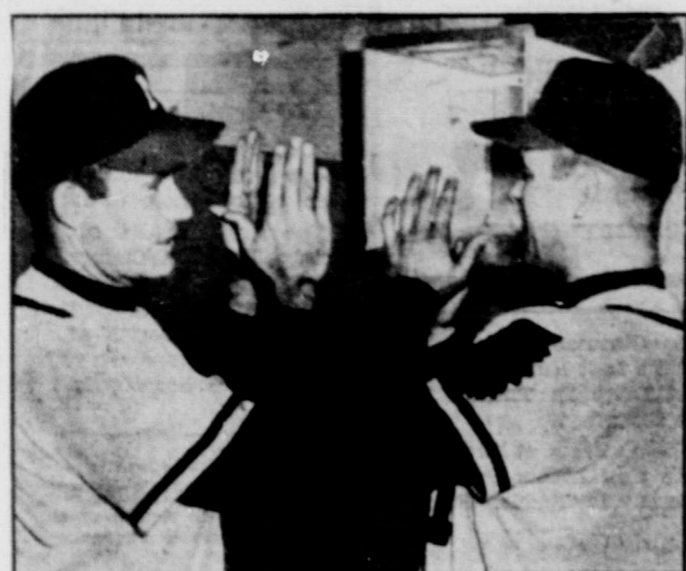
HOT TIME IN THE DUGOUT —Milwaukee Braves' first baseman Joe Adcock, left, and third sacker Ed Mathews warm their hands at an infrared heater in the dugout of Milwaukee County Stadium. Installation of the devices is one of the first in a United States sports facility. Designed for outdoor use where heat can be focused at a desired spot without an attempt to heat all outdoors, the infrared heaters have found wide spread use in Europe at outdoor restaurants and sports stadia.
