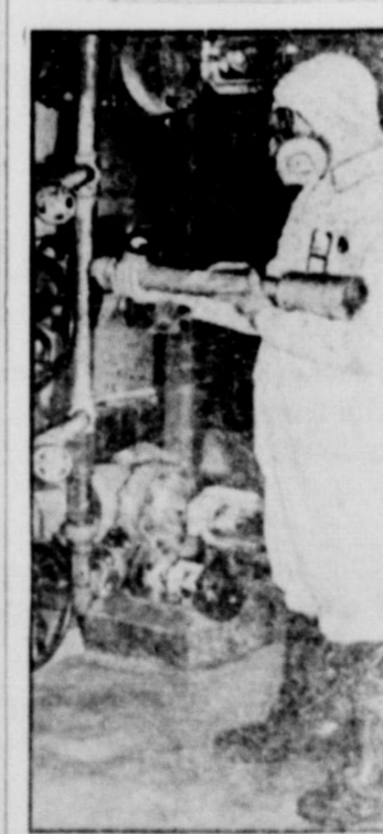
ATOM-AGE PLUMBER —Technician at the Hanford Atomic Products Operation, Richland, Wash., carries a meter instead of a monkey wrench when searching for leaks in "hot" plumbing. The GE-developed device employs a sodium iodide crystal, light output of which under atomic radiation is measured on a light-type meter at end of barrel.
