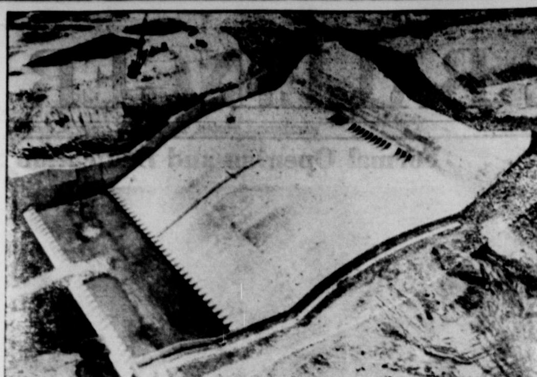
MONEY IN THE TILL —That's what water from cash register-like spillway means to neighboring farmers of Kirwin Dam, near Phillipsburg, Kan. The recently completed key unit of an 11,500-acre irrigation project, dam is 12,616 feet long, has a 400-foot-wide spillway and cost $19,500,000 to build.
