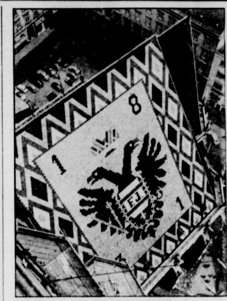
FREEDOM UNDER THE DOUBLE EAGLE —Coat of arms of the former dual monarchy of Austria-Hungary and also of the House of Hapsburg once more glitters over an Austria which is once again independent of both royal reign and occupation. Workers have just finished restoring the half-million-piece tile mosaic on the roof of St. Stephen's Tower, Vienna, which was destroyed by fire in 1945.
