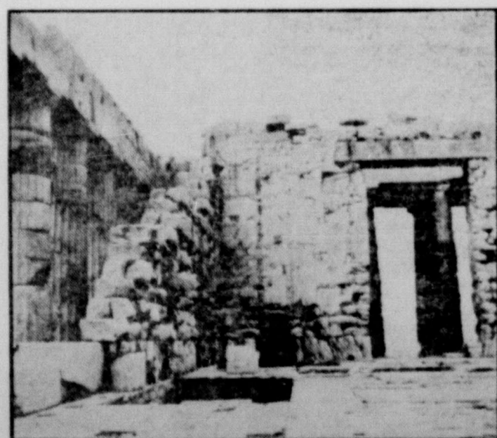
TEMPLE TO BE ROOFED —The Greek Archaeological Council will soon erect a roof over the ruins of the Parthenon, to protect the ancient Greek temple's sculpturing. The inner walls, such as the one shown to the right of the columns, will be demolished in hope of discovering ancient inscriptions of archaeological interest.
