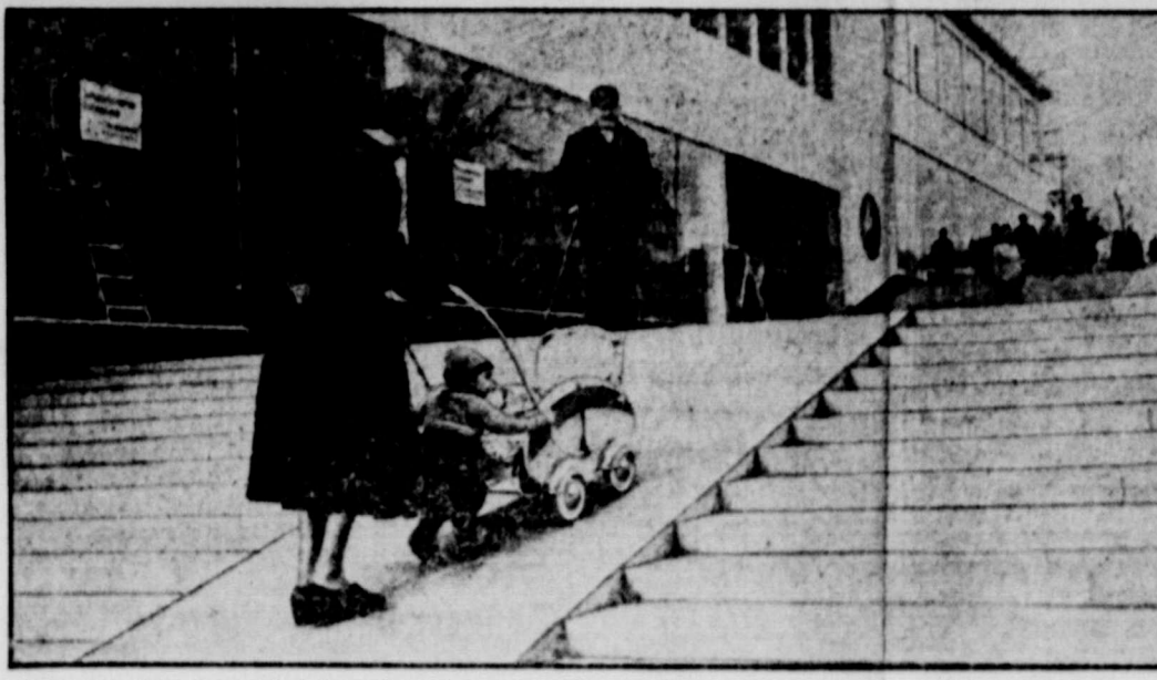
STAIRCASE STREET—This new street in Kassel, Germany, is just one big staircase—for pedestrians only. Approximately 90 yards long and seven yards wide, with a runway for baby carriages up the middle, the street was built at a cost of some $47,500.
