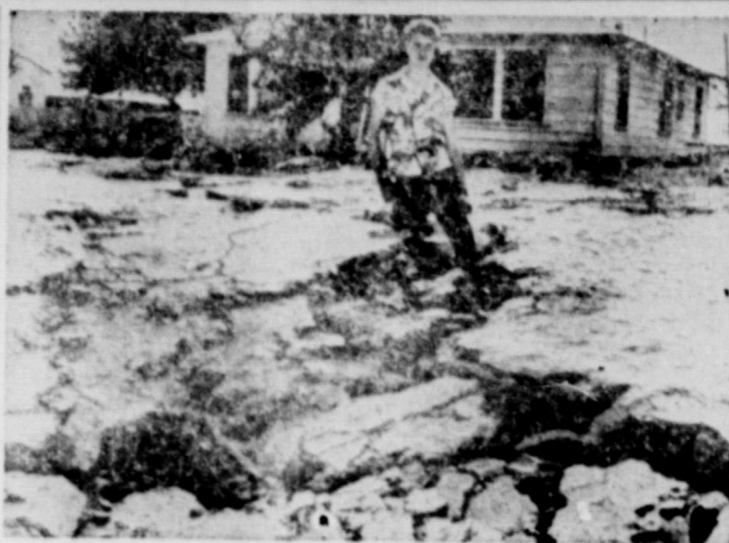
CALIFORNIA QUAKE . . . Jack Garren, 14, stands knee deep in a great crack left in the ground by repeated earth tremors in Arvin, California, recently. Continued earth shocks have added to the already huge toll in property damage since the original earthquake. Arvin is near Tehachapi which the great quake practically demolished. Property damage has been estimated in the millions of dollars. Eleven persons were reported killed. Numerous minor shocks have been recorded since the disastrous original quake.
