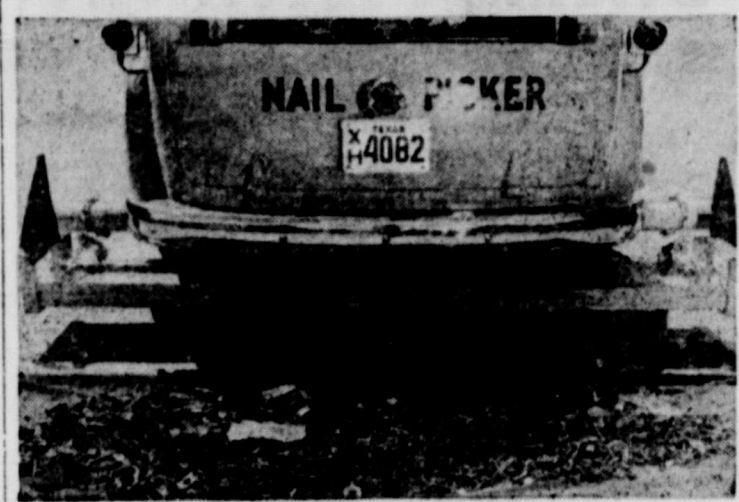
The magnetic nail picker of the Texas Highway Department will arrive in Runnels county soon to sweep the highways and road shoulders of all metal objects. Electric magnets at the rear of the nail picker collect loose metal objects. The magnets are activated by a large generator in the bed of the truck and are strong enough to pick up manhole covers. In the pile of scrap metal above are some 2,000 potential punctures.
