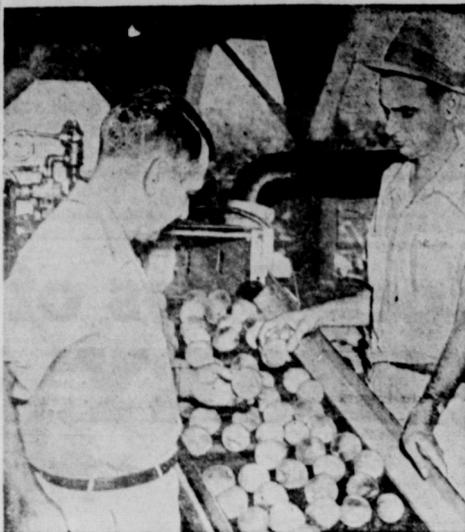
**CLEAN-SHAVEN PEACHES** . . . Soon, thanks to this machine being tried in Spartansburg, S. C., your peaches will come to you in shifting nudity. The gadget is a peach polisher designed to take the fuzz off the peach and apply a thin coat of wax to seal in the natural flavor of the fruit and reduce shrinkage. Revolving brushes do the job. Examining some newly-shaved peaches as they come through the machine are Les Collier and Ben Gramling. No, an electric razor won't work.
