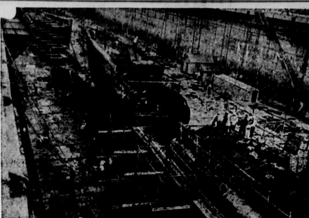
STRETCHING THE REDFIN . . . United States navy workmen are pulling apart sections of the hull of the U.S.S. Redfin, the undersea craft being lengthened at the U.S. naval shipyard in Philadelphia, Pa. A new middle section is in preparation to be fitted into the gap left by the workmen to make room for some vital new war equipment which is so top secret that naval officials will not disclose what is the function of the equipment in sea warfare. However, certain officials have been authorized to state that the submarine, when repairs are completed, will become an entirely new type of undersea weapon, never used in war before.
