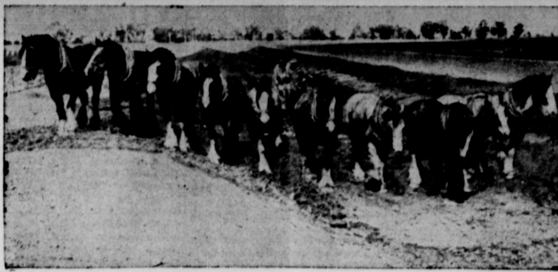
TEN HORSEPOWER IN ACTION . . . In these days of power-driven machinery, a ten-horse team is as rare as that day in June. This team is in use building an irrigation canal in the Murray valley soldier settlement, Victoria, Australia, where between 500 and 600 miles of irrigation channels are being excavated. The horses are used in preference to power machines because stamping of the horses' hoofs helps bind the soil on the banks of the channels. Notice the size and weight of the horses in this team. No wonder their feet bind the soil.
