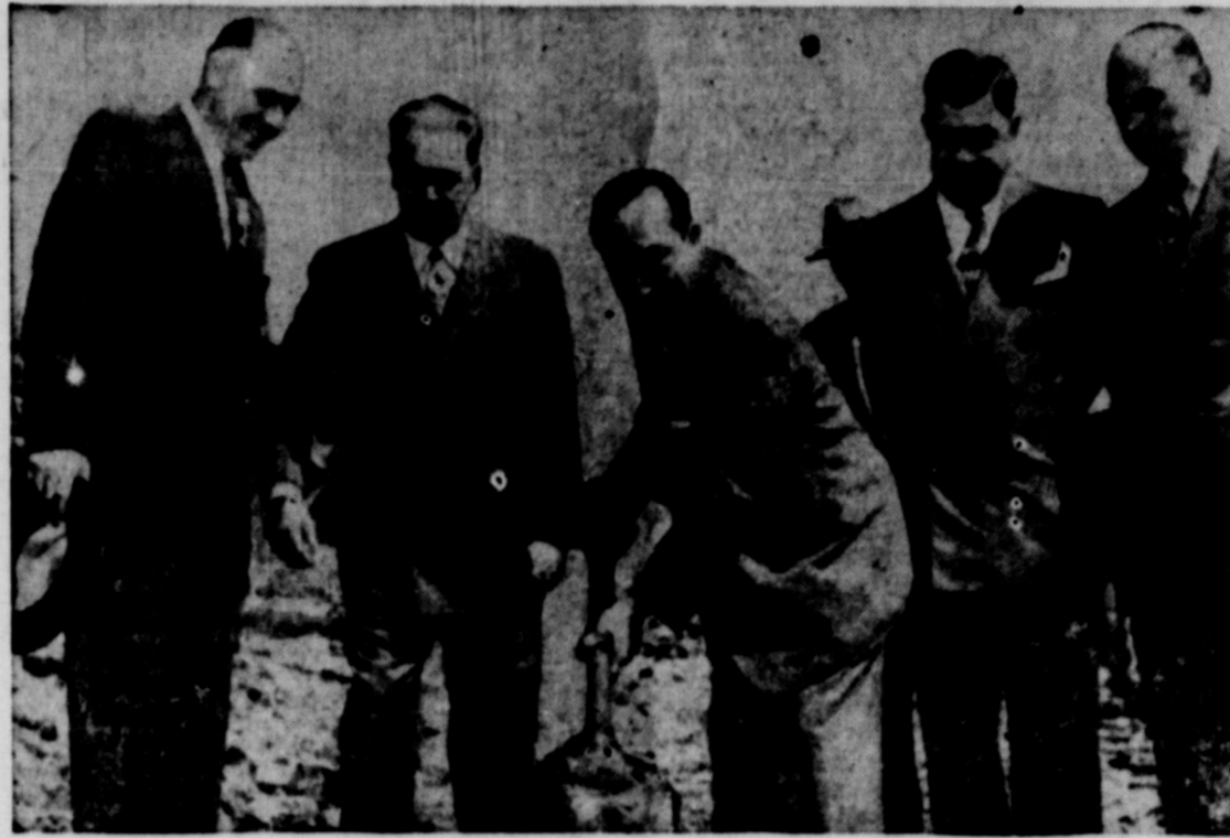
BUILDING A MONUMENT TO PEACE . . . Benjamin F. Cohen, acting secretary of the United Nations, takes the first shovel of earth from the site of the United Nations' permanent home on New York's East River site. Cohen is hopeful that this "world capital" will succeed in maintaining peace. A $65,000,000 loan for the construction of the building was approved by congress and the building now can proceed. In the ceremonial group are left to right: Hugo Rogers, borough president of Manhattan; Mayor William O'Dwyer, Cohen, City Comptroller Lazarus Joseph and Deputy Mayor John J. Bennett.
