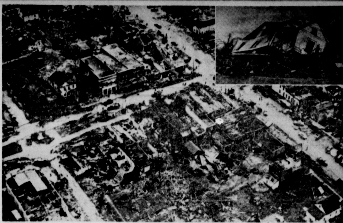
SHATTERED BUNKER HILL . . . The word "tornado" invariably calls to mind two accompanying descriptive terms, "death and destruction," and in the case of the twister that howled through west-central Illinois those adjectives were as appropriate as ever. It cut a furious swath through an area 50 miles wide and 100 miles long, leaving behind a death toll of 31 and a trail of shattered residences. Hardest hit community was Bunker Hill, almost completely destroyed by the force of the tornado. Inset shows a closeup of one of many houses that were shattered like cardboard toys.
