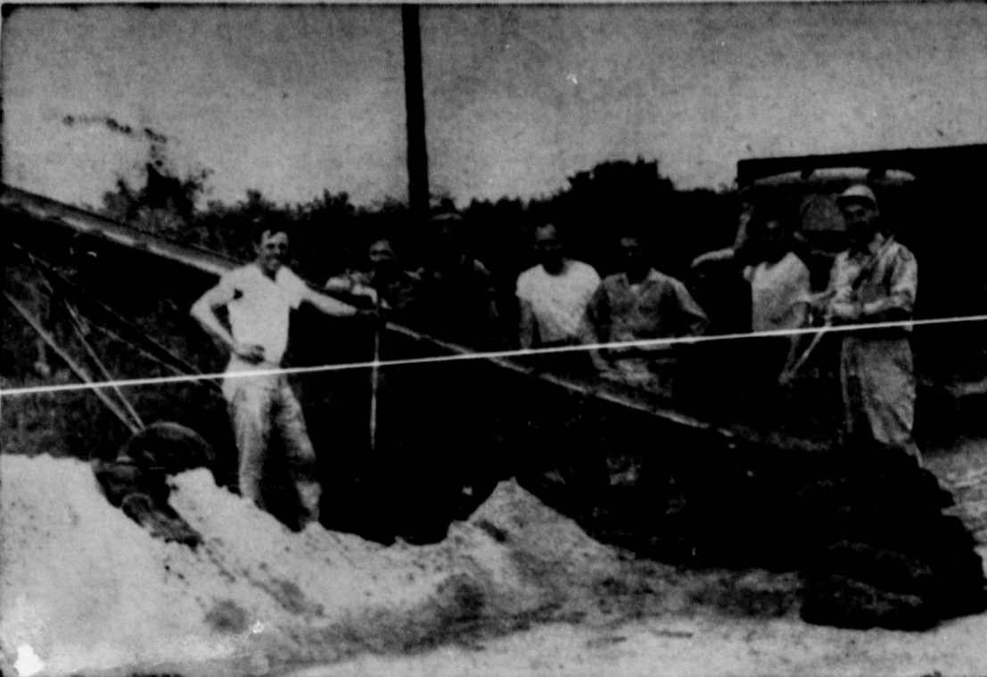
'KNOW-HOW' HELPS DEFEAT FLOOD MENACE . . . With the Mississippi off on one of its most destructive benders in a century, farmers up and down the river were hard put to keep the rampaging waters from flooding their fields. At Wapello, Ia., this crew of flood fighters rigged up a portable grain elevator to carry sandbags up to levee in background for speedier reinforcement and to eliminate necessity of workers' hauling heavy bags up the slippery 15-foot embankment.
