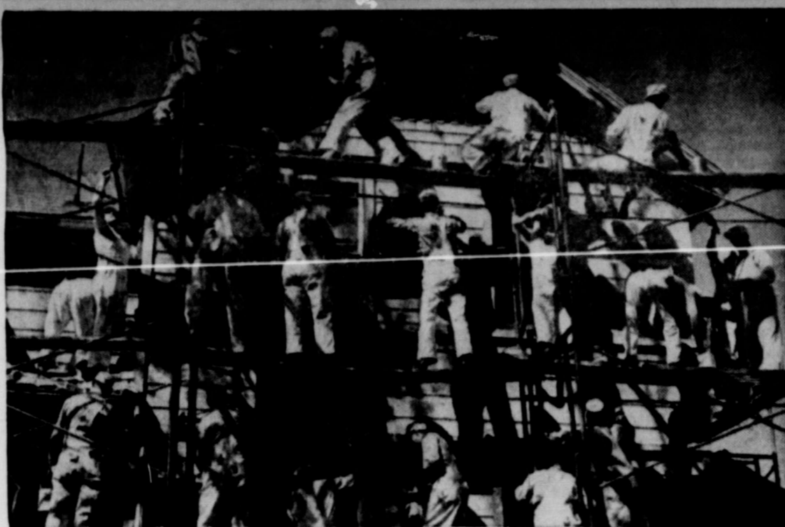
SO IT'S NOT IMPOSSIBLE . . . There was a great flurry of brushes and pigment as 100 painters in Salt Lake City ganged up on a two-story, seven-room house and painted it—including trimming for windows, eaves and doors—in nine minutes and seven seconds. The stunt was part of the civic beautification program for Utah's centennial celebration and it resulted in a new record for a fast brush-off.
