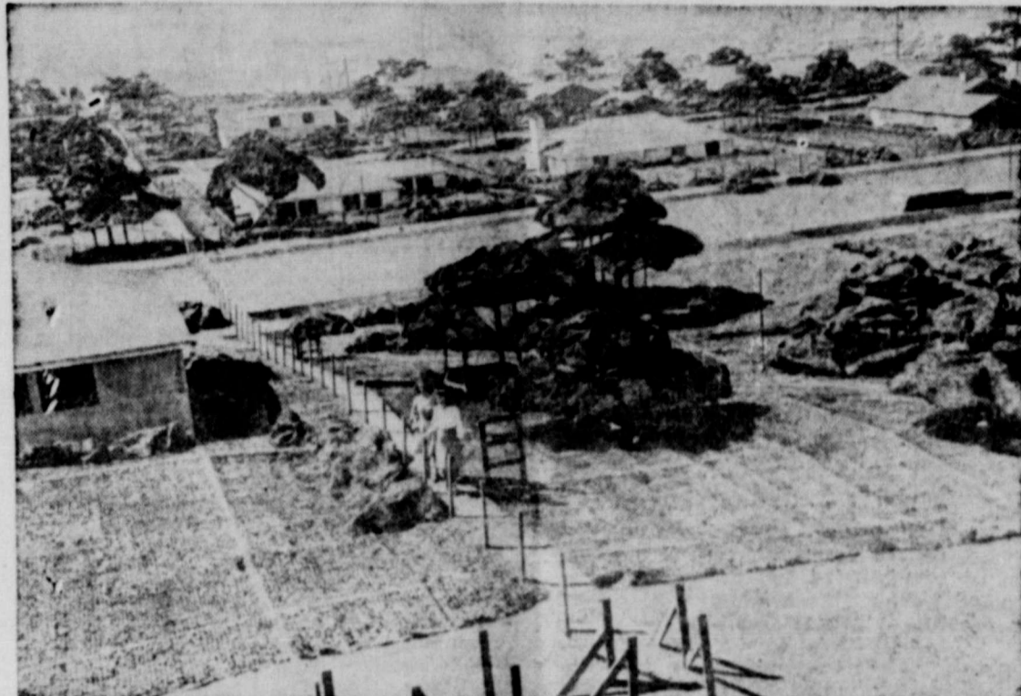
This peaceful village isn't—it just doesn't exist—look again, closely this time. You can see that the houses only look like houses and the trees are strictly imitation. About the only real things here are the girls, Suetelle Lamoreaux and Elmer Offenbach, who use a "safe" catwalk and stay off the chickenwire farmland of this elaborate camouflage which has been built to protect a vital B-29 plant from threat of possible Japanese air raids. This is the first photograph of this camouflage project—the top of a factory!
