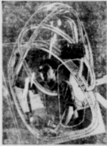
This "Lucite" crystal-clear nose of a Martin bomber is one of the largest plastic pieces ever manufactured on a mass production basis. An essential ingredient in plastics for war use is used kitchen fat.
