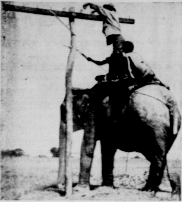
A member of the American signal construction outfit is shown repairing a line from the back of an elephant. These slow-moving, patient animals are used to very good advantage in the swamplands of Assam, India, by native and Allied troops. The signal corps, under unusual conditions, have managed to install and keep open communication lines.
