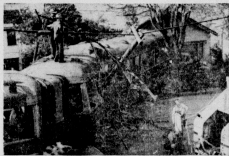
After hitting a piece of concrete on the rails, this train jumped its tracks, crashed into a steel trolley pole and careened 29 feet across a street, stopping only two feet from the home of Oscar Houman. He later said he thought the noise was an earthquake. The accident occurred in Berkeley, Calif. Seven passengers received minor injuries.
