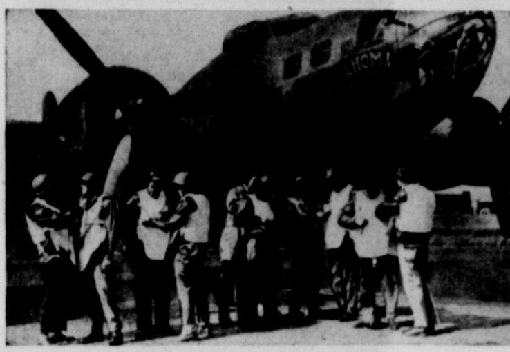
Members of a crew of a Flying Fortress are shown helping each other don their armored flying vests at a United States bomber station in England. Made of tough manganese steel, these vests protect the airman from flak shrapnel and fragments of cannon shells. A quick pull on a rip cord causes the vest to fall away from the body.
