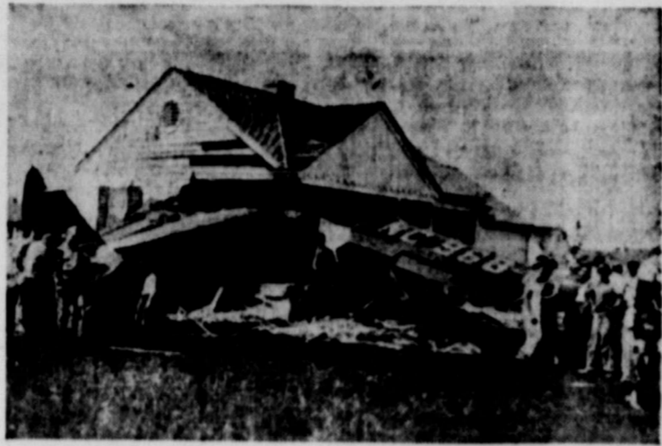
This WAS a house! And that WAS a plane sticking out of the shattered timbers. Spectacular picture, taken just after the plane ripped into the side of a cottage near Glenview, Ill., shows graphically the aftermath of the crash. Four passengers were only jarred when the plane, en route to Mexico, hurtled down to earth after the motor suddenly failed.
