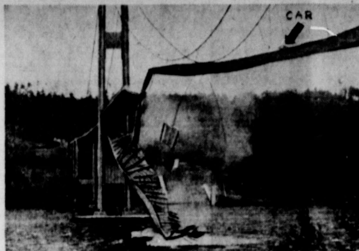
This soundphoto shows the new Narrows bridge at Tacoma, Wash., third longest single suspension span in the world, as it started to disintegrate and fall 190 feet into Puget Sound. The bridge was completed last July at a cost of $6,400,000. Note the car on the bridge which was abandoned by its occupants as the bridge began to collapse.
