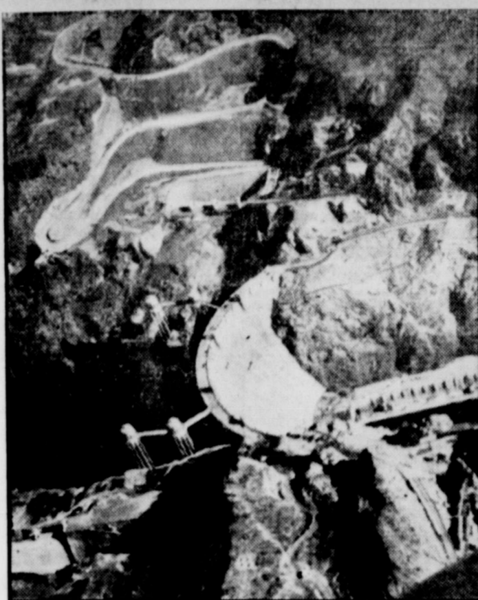
At first glance, this scene appears to be a view from above of China's winding, historic Great Wall. But in reality it's an air view of America's Boulder dam and lake. The Great Wall effect is created by a new serpentine roadway leading from the dam to points in Arizona.
