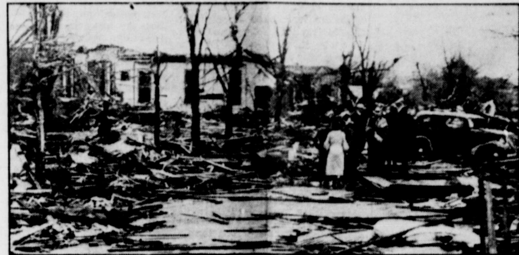
This scene of complete ruin in Tupelo, Miss., was typical of the desolation to be found in many other towns after record tornadoic winds swept across eight southern states. The dead in Tupelo alone numbered more than 200, with property damage set at about $5,000,000. The complete death toll exceeded 500. City officials estimated that it would take at least 10 years for Tupelo, a town of 8000 in northeastern Mississippi, to rebuild.
