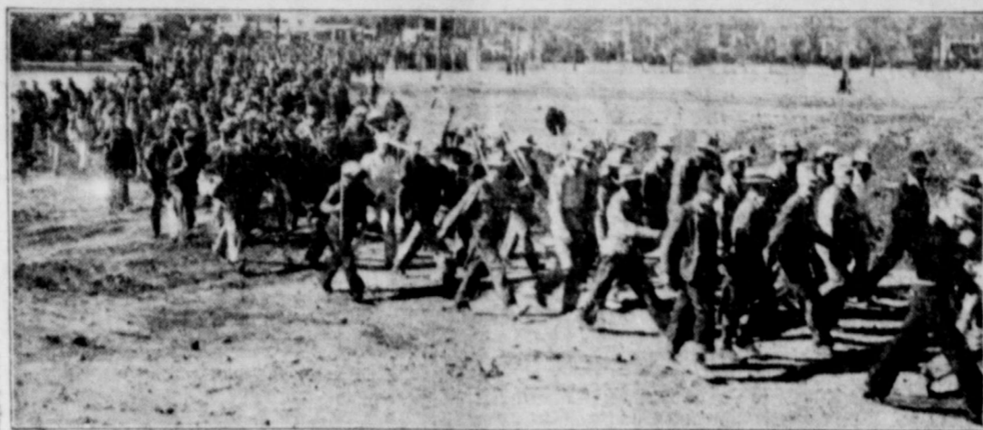
Three thousand men are working each day on the huge lot of the Texas Centennial Exposition in Dallas. Three shifts a day speed work for the opening date, June 8. Above workmen are shown filing in for the late afternoon trick. As the Exposition, federal, state, city and exhibitors' building schedules develop, more men are hired daily, further cutting into the fast vanishing ranks of Texas' unemployed.
