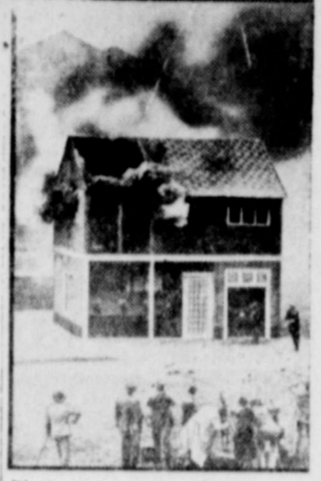
Blasts are so often the cause of fires, that it's news when explosions are employed to end them. This London conflagration, in a test, was extinguished in four minutes by means of chemical-filled cardboard bombs set off by the heat.
