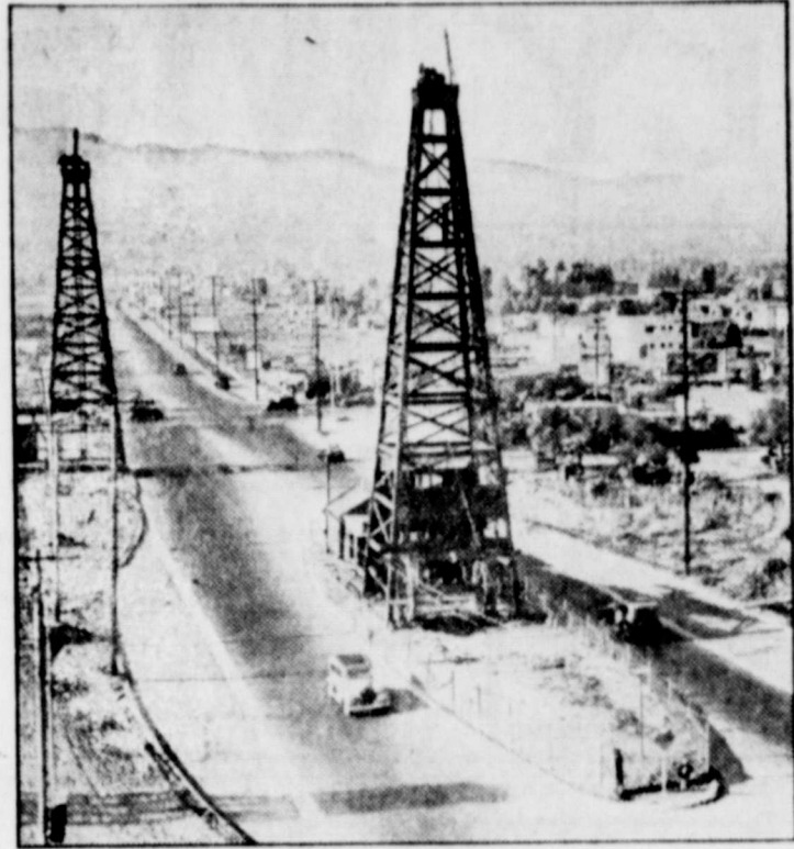
Out west, where oil is king, wells spring up in the oddest places. In Oklahoma City they crowd downtown skyscrapers; here, in Los Angeles, discovery of oil beneath a thoroughfare made necessary the creation of this street "island," from which an oil tower juts.
