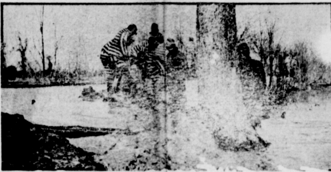
Convicts from the Mississippi state prison trying to stop a break in the Coldwater river as flood waters pour through. The floods along the Mississippi have caused property damage estimated at $5,000,000 and rendered some 25,000 persons homeless and destitute.
