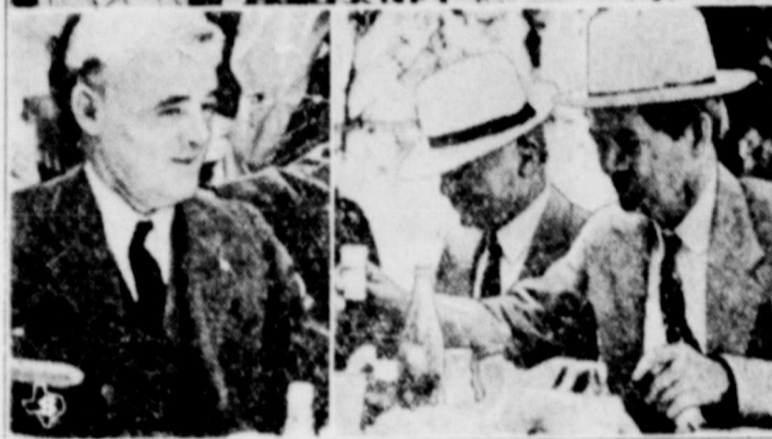
Above is a view of the half-finished Buchanan Dam on the Colorado River above Austin, Texas, which may be completed soon if the Colorado River Authority program is passed by the Texas legislature. Below are shown Henry T. Hunt of New York (left), who represented the PWA at a recent "get-together" at the dam. He said the PWA favors completion of the dam because it means modernizing many Texas farms with canal electrification. Farther lower right is Congressman James P. Buchanan after whom the dam was named. The pictures were taken at the party at barbecue at the Hill country between Llano and Burnet. (Texas News Photos.)
