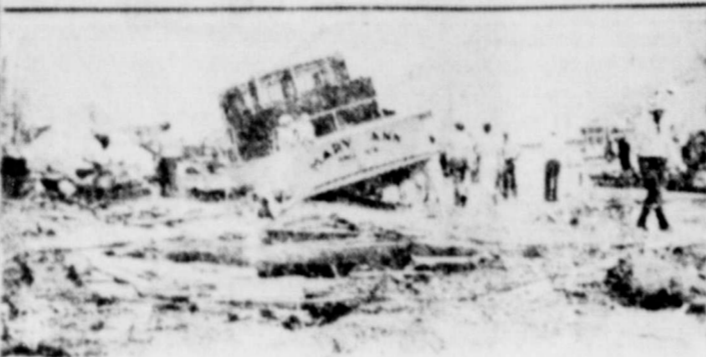
These pictures from Port Lavaca show some of the havoc wrought by the storm that recently visited the Gulf Coast. Buildings were damaged by wind and wave and many boats were carried inland and damaged. (Texas News Photos.)
