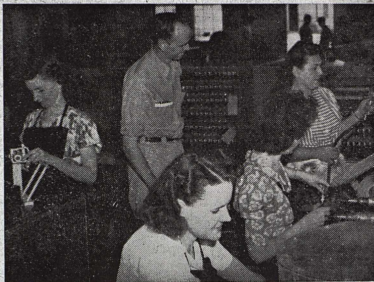
The above picture shows five members of the spark plug maintenance department at work. Left to right: Mrs. Myrtle McKenzie operates a rethreading machine; Mr. James W. Horton, department foreman, supervising operations; Mrs. Wanda Tittle, sand-blasting plugs; Mrs. Hazel Epperson, using buffer to remove rust; and Mrs. Jeanette Whaley, spraying plugs to remove rust. Two members of the department not shown are Mrs. Beatrice Dickerson and Miss Lois DeMasters.
