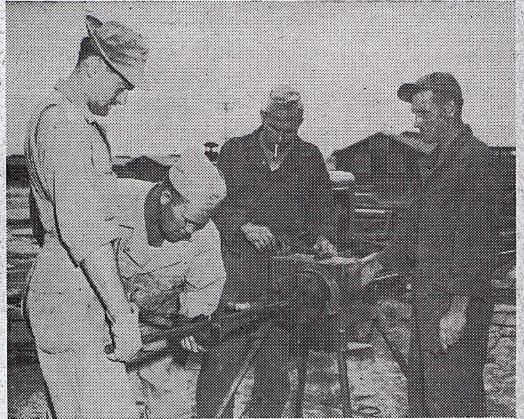
Cutting some small joints of pipe for fitting is this group. Left to right: Pvt. Glenn Caughey, Pvt. Verne Pinney, S-Sgt. Thomas J. Smith, and Sgt. Delbert Simpson.
