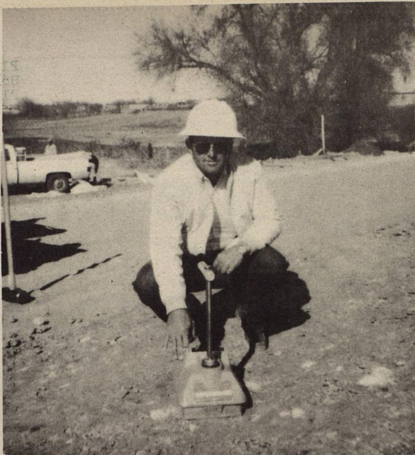
AT WORK ON SH 214 - Gary Smith, engineer technician with the State Highway Division of Texas, is shown taking compaction density with a nuclear density guage in fill north on 214. A native of Plains, he is the son of Amos and Doris Smith. Construction on 214 is being performed by Ivan Dement Construction.
