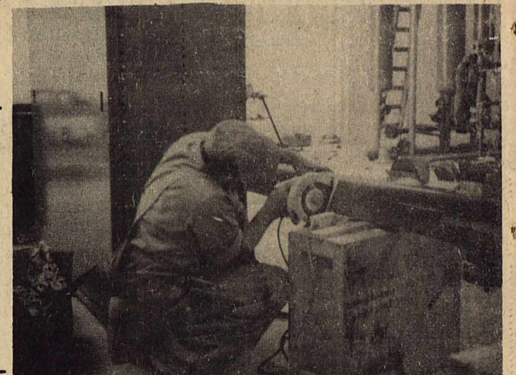
Workman at construction of "Permasap" plant.
