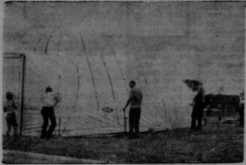
UP IT GOES is the word, as the unusual tent in which the Santa Anna Seventh Day Adventist Church will hold its two week long revival beginning next Saturday, is erected by a volunteer crew. The tent needs no poles to hold it up, being supported entirely by air pressure.
