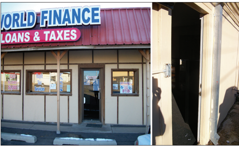
Submitted photos The World Finance building located at 1534 N. Hobart St. The photo on the left shows the back door where the perpetrators broke into the building and stole electronic equipment and cash.
