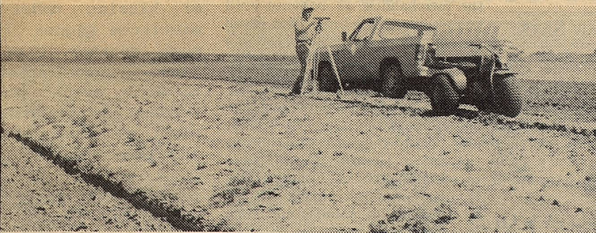
Buddy Watson, District Technician, is shown checking ACP terraces on the Doyle Newton ranch in Borden County. The construction of terraces and diversions is an excellent way to control and stop erosion on rolling land and sloping cropland. With terraces and diversions, rainwater is channeled across the field to a suitable outlet such as a grass waterway or pond. Through this channeling action, water is transported across the field and isn't allowed to cut down across the field, stopping erosion and the development of gullies.
