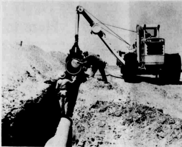
AFTER DELAY, WORK CONTINUES--Workers were moving on toward the sandhills with a 24-inch city pipeline this week after a legal hassle had slowed the project Friday and Saturday. Shown here is a big side-boom rig which is used to lower the 30-foot lengths of pipe into the ditch.
