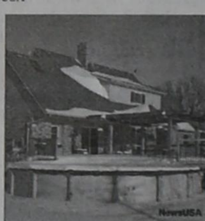
Improperly winterized pools can sustain damage to equipment and underground drains - damage that can cost thousands to repair.
