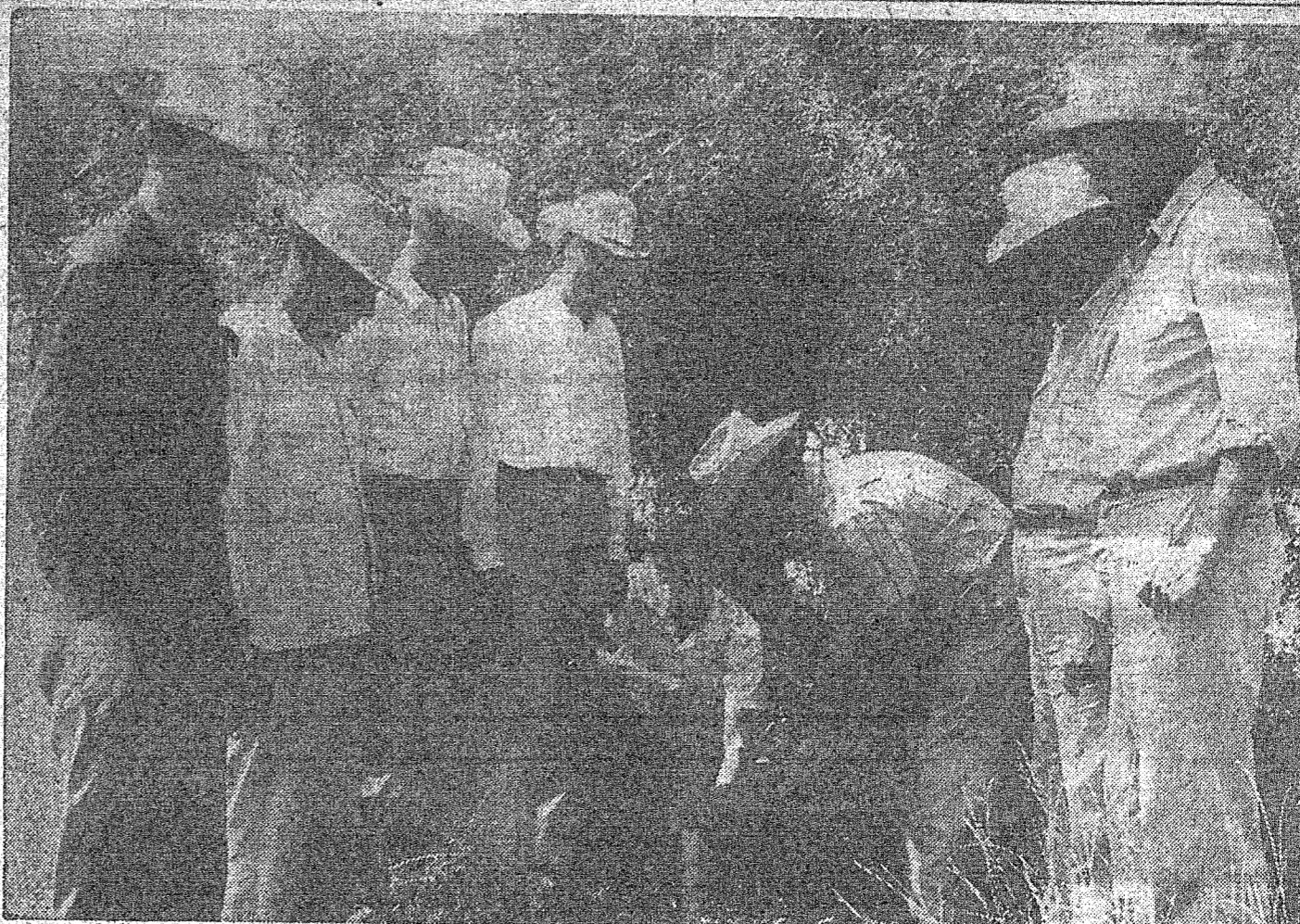
FIRST TELEPHONE STAKE — Raymond McElrath of Coleman, president of the Coleman County Telephone Cooperative, Inc., bends over to drive the first stake for the new rural telephone system which is in the process of being installed in the southern part of Coleman County. A 450 mile area will be staked for telephone lines running from Santa Anna to Trickham, Rockwood, Valera, Flsk, Gouldbusk, Leaday and Voss. The Shields and Whon area will be on the Rockwood switchboard. Directors of the Cooperative are, left to right, R. A. Powell, vice president, Fisk; S. S. Squyres, Gouldbusk; Uless Maness, Rockwood; Frank Gillespie, secretary, Coleman; Jack Covington, engineer, Abilene; President McElrath; Emzy Brown, Santa Anna, and J. D. Gorman, Novice. George M. Johnson, Santa Anna, not pictured, is the local manager of the co-op.
