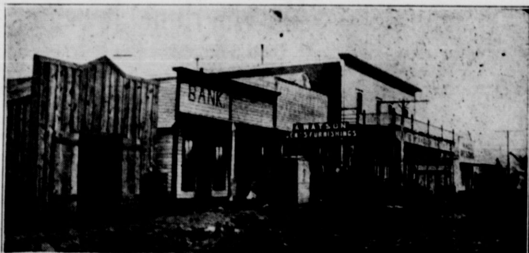
SOUTH SIDE of Dundee Street facing the courthouse square about 1905. Buildings from left to right are: A. Kanzler's blacksmith shop, Matador's first bank; A. Watson's men's clothing; Van Martin grocery; Chalk hardware company; and Matador Mercantile, operated by Jack Luckett. The blacksmith shop is about the present site of the Matador post office.
